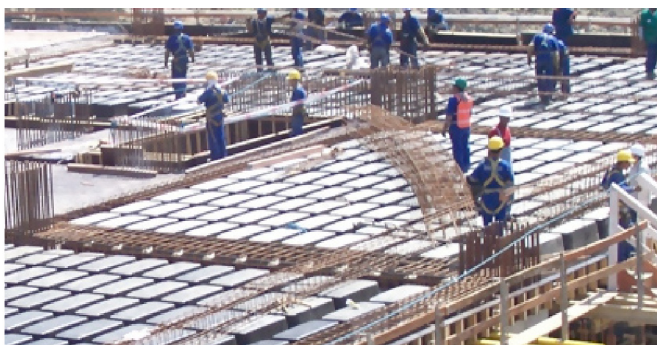
Figure 3 – Construction Process using ATEX molds Source: ATEX (2012)
